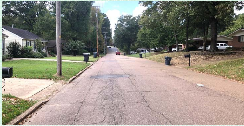
Incomplete Street: driving lanes only
