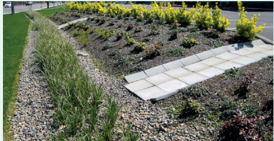
Bioswales filter and retain stormwater run-off.
