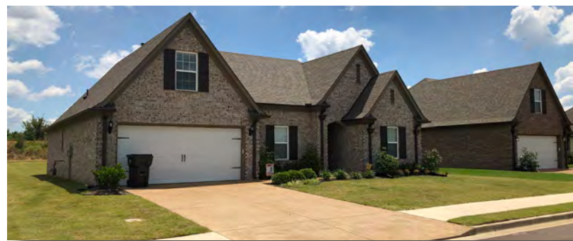
The largest percentage of Hernando's developed areas are occupied by single-family neighborhoods. Those developed during the past few decades are very auto oriented with garages and driveways dominating their streetscapes.
