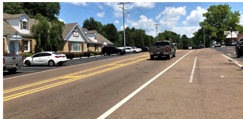
This segment of Hwy. 51 near W. Northern Street illustrates some of the access management issues that exist in Hernando. Both sides of the street lack sidewalks and a landscaping strip. In fact, drivers on the left side of the street are forced to back out directly onto the street.
